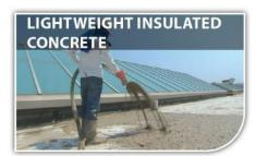
Lightweight concrete delivers many new benefits that make it an excellent alternative in roofing today. Its ability to provide high insulation values with reduced weight, reduced costs during installation and re-roofing, and a lower impact on the environment all make lightweight concrete a superior choice.
